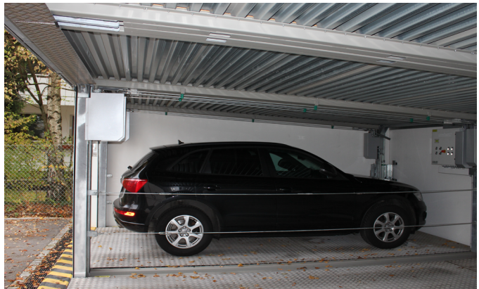
Systems with mobile roof seen from the side
