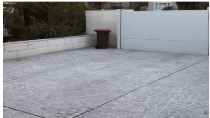
Synthetic stone covering (3 cm thick)
