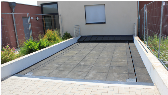
Rubber covering in stone structure (3 cm thick)
